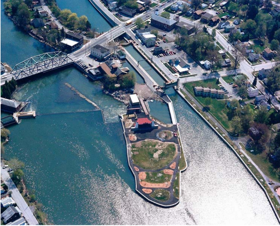
Picture reprinted with permission from Plumley Engineering, Baldwinsville, NY
